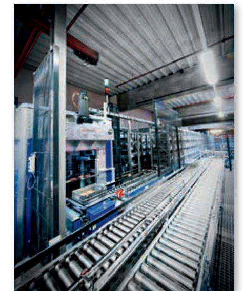
Perfectly networked. Our long conveyor system brings the items included in an order to the correct packing station.
